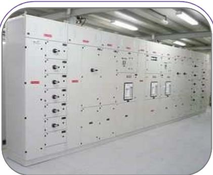
LV panel boards & switchgears
